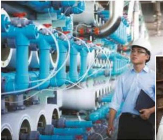
Reverse osmosis membranes used in the production of NEWater.
