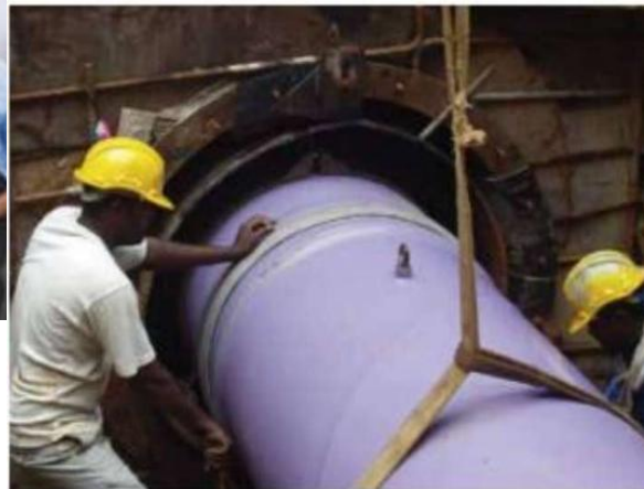
NEWater pipes are built to meet the demand for NEWater.
